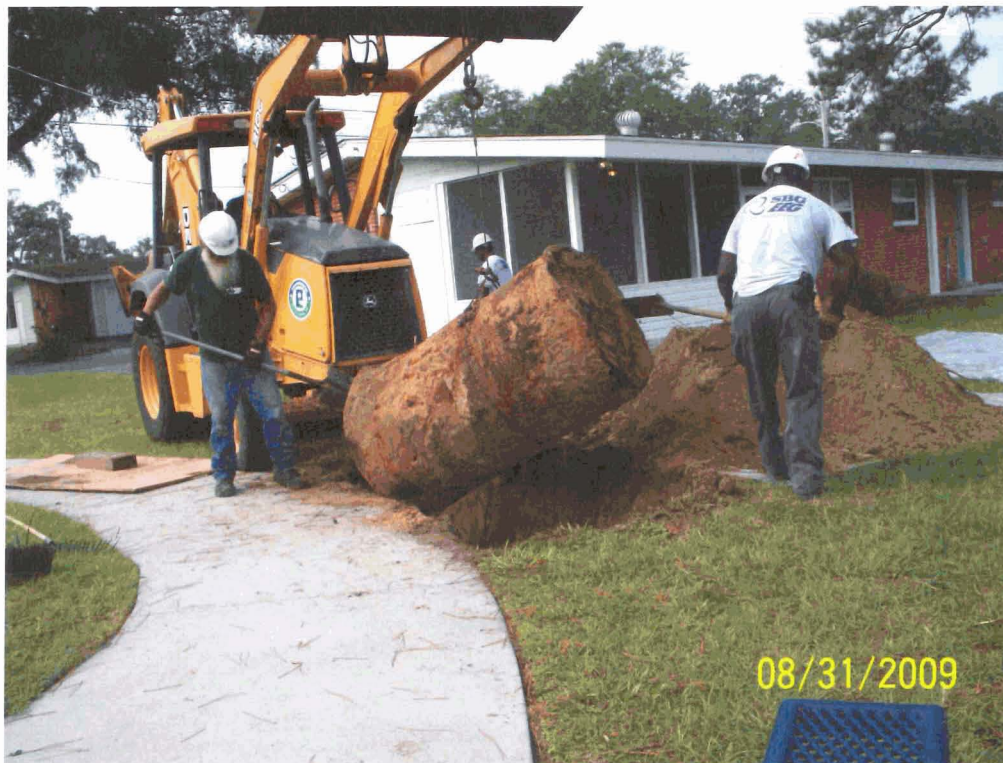
Picture 2: UST 1247Dove removal in progress.
